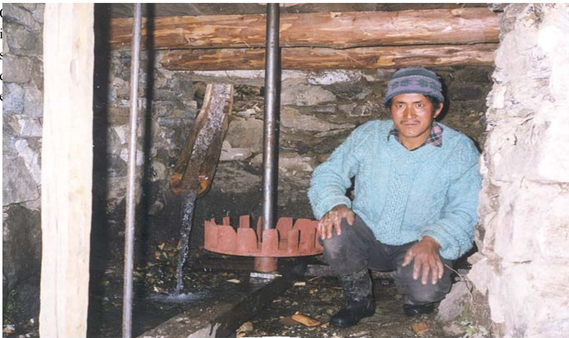
Improved watermill runner being installed in a village in India
