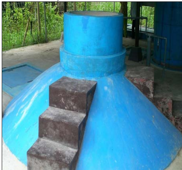
Figure 7.8. A fixed dome small scale biogas digester for a household uses introduced by Muhamadiyah University, Malang, East Java Province, (Source : DEMR)
