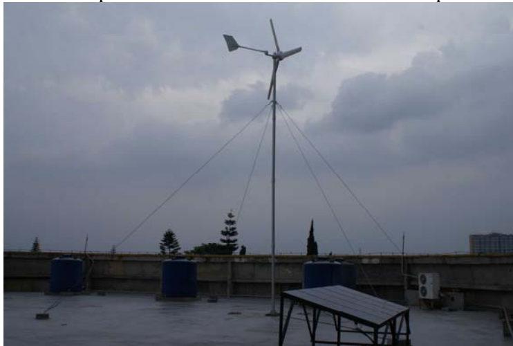
Figure 7.6. Installation of a 2.5 kW Wind Power Electricity Generation unit, an example of DEMR activity on RE at Sukabumi, West Java Province.
