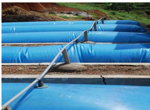
Figure E : Simple biogas collector to collect gas for electricity generation in rural area.
