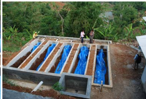
Figure E : Simple biogas collector to collect gas for electricity generation in rural area.
