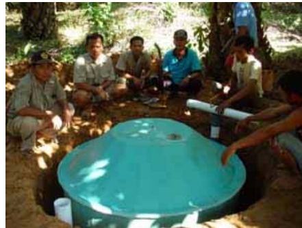
Figure C : A typical digester, for a company, PT. Asian Agri , in Jambi Province, to be utilize for electricity generation for local households.
