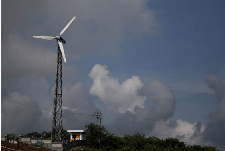
Figure 7.7. Wind Power electricity Generation, 80 kW system, at Nusa Penida, Bali built by DEMR (Source : http://daus.tral.la/2007/12/nusa-penida ).
