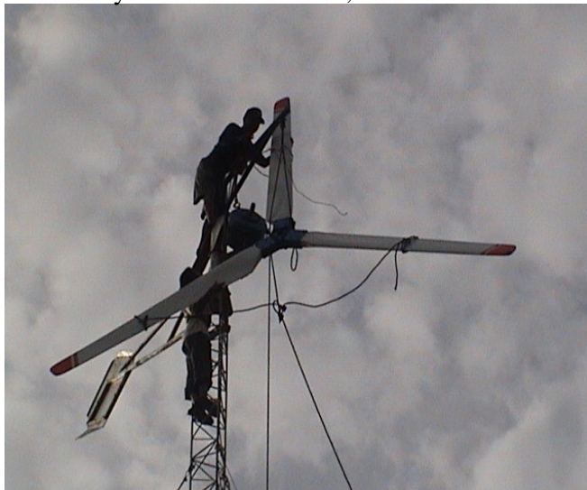
Figure 7.6. Installation of a 2.5 kW Wind Power Electricity Generation unit, an example of DEMR activity on RE at Sukabumi, West Java Province.
