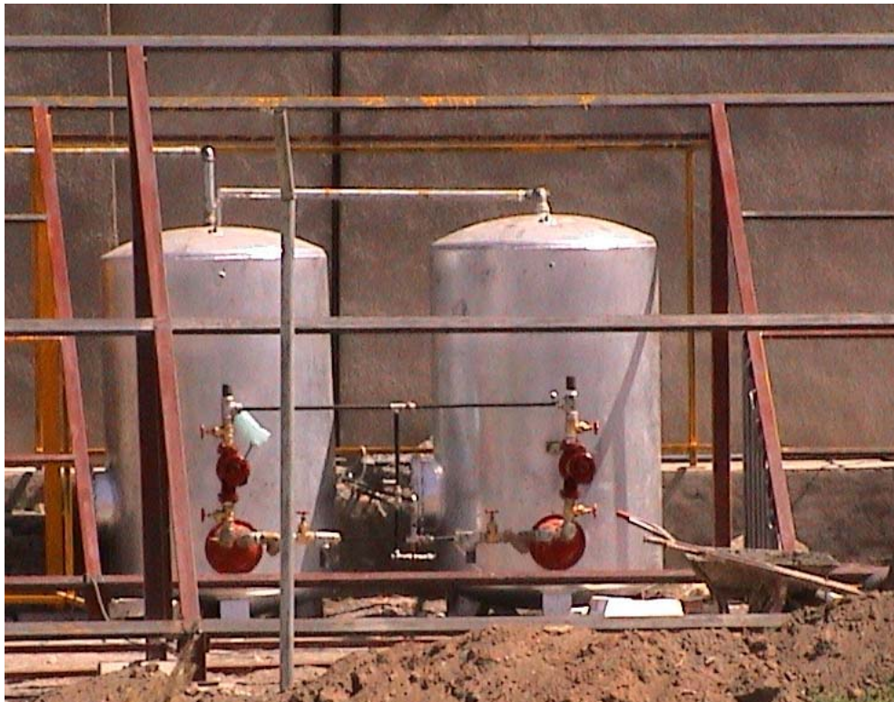
Fig. 8.21 Two storage tanks under the structure
