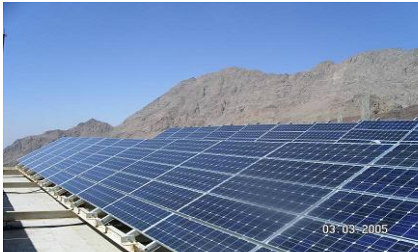
Fig.4.11 Five KW e photo voltaic system near the Yazd
