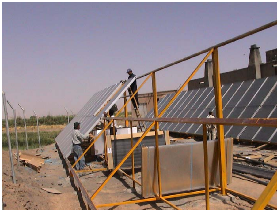
Fig. 8.19 Installing solar collectors
