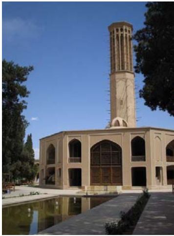
Fig.6.1 wind tower in the city of Yazd
