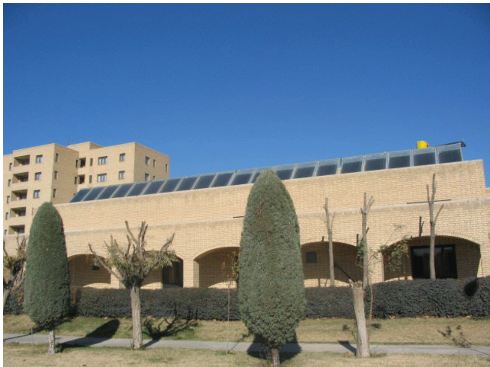
Fig.8.2 Solar collectors building
