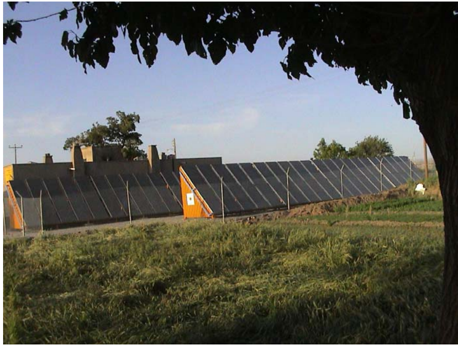
Fig. 8.22 System is completed
