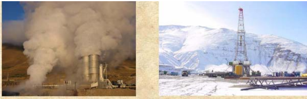
Fig.4 18 Geothermal power plant with final capacity of 100 MW in vicinity of mountain Sabalan
