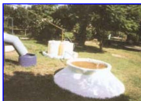
Figure 8.13 – Batch Type Lankan Biogas Generator (Source: - NERDC)
