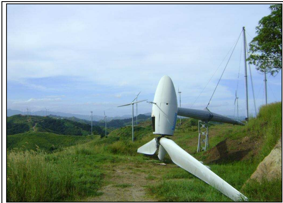
Butoni wind farm during its construction stage in 2007
