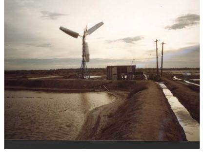
Figure 4.1 Water pumping windmill installed on the banks of salt pans
