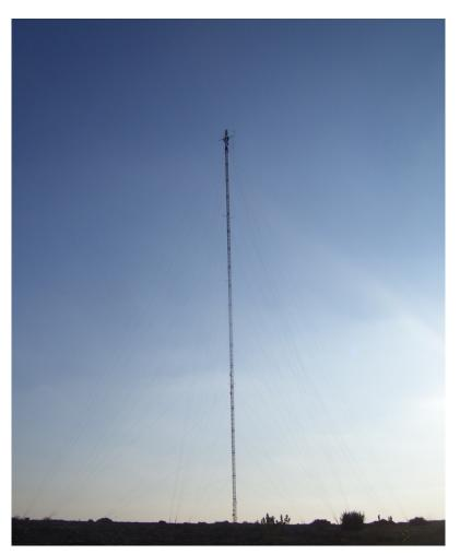
Figure 2.2 A typical wind monitoring mast.
