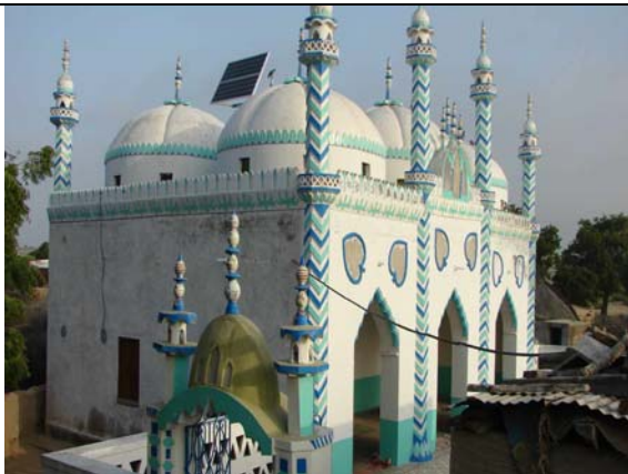
200 Watts Solar Powered System at a Mosque in Thar Area
