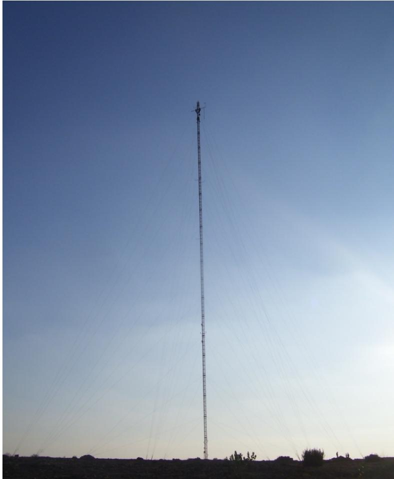
Figure 2.2 A typical wind monitoring mast.
