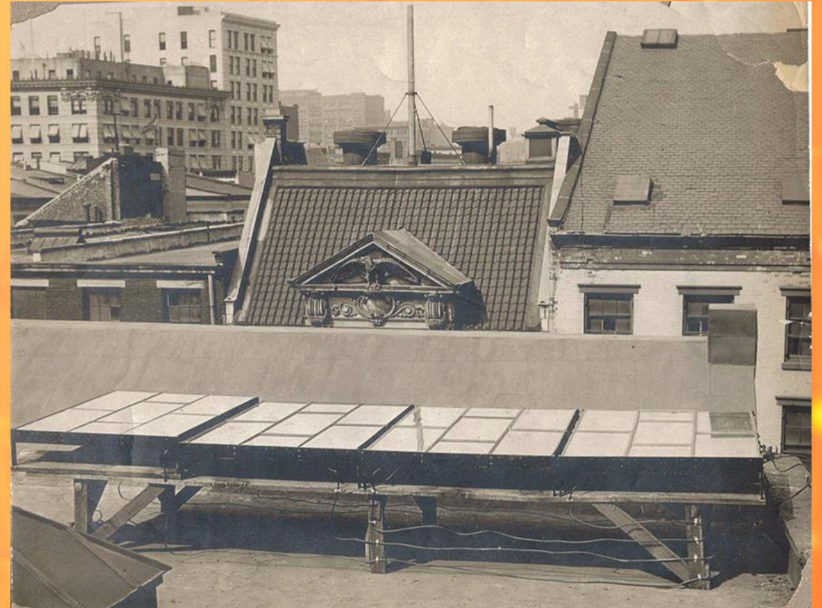
▲ Charles Fritts installed the first solar panels on New York City rooftop in 1884
