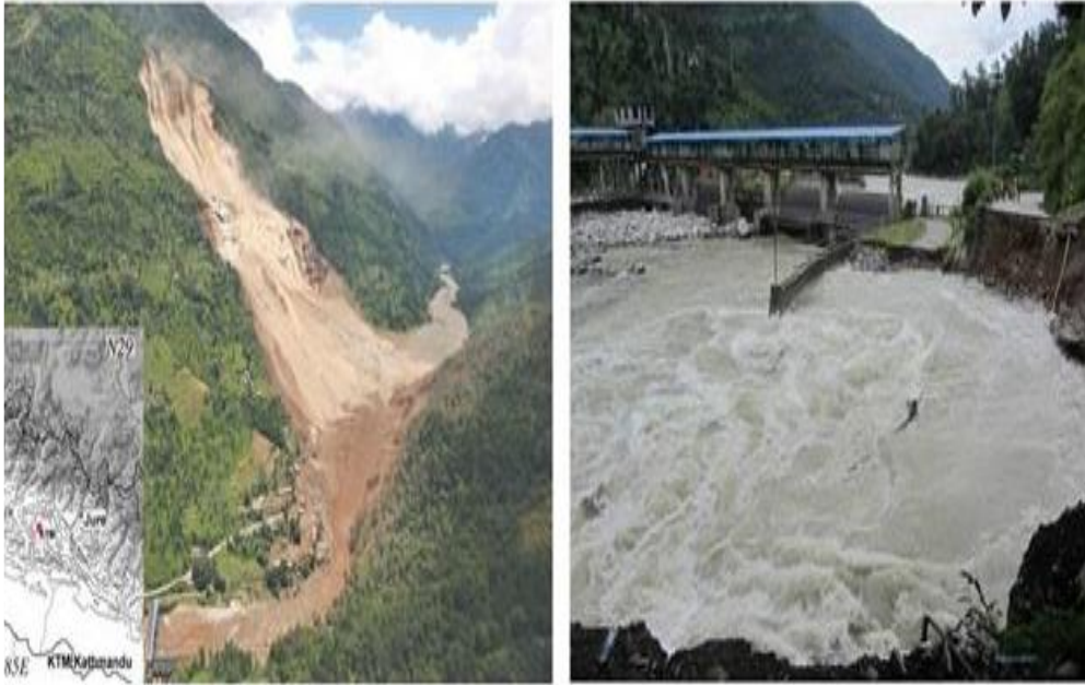
Sunkoshi 10.05 MW Power Plant : 2014 - Jure Landslide caused by heavy rainfall dammed the Sunkoshi River and caused severe flooding downstream on breaching of the dam.
