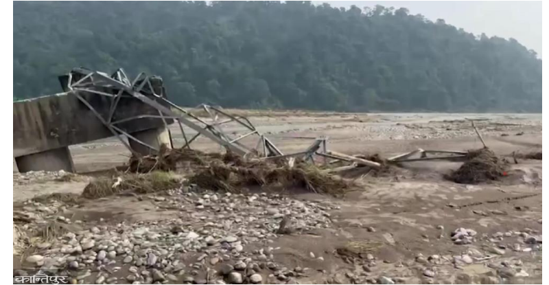
Wreck of transmission line structure (Kabeli Corridor: 200 MW)
