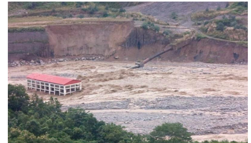
Submerged power house (Bagmati Small Hydropower-22 MW)
